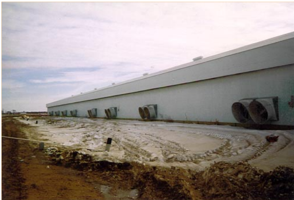
Layer house with 'deep pit' Ventilation
